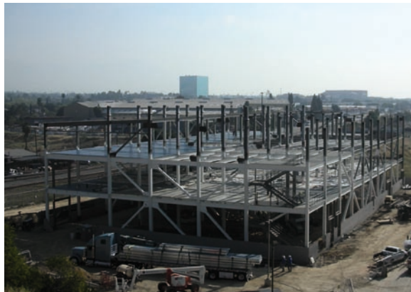
Construction of the new IGIV plant in Los Angeles.
